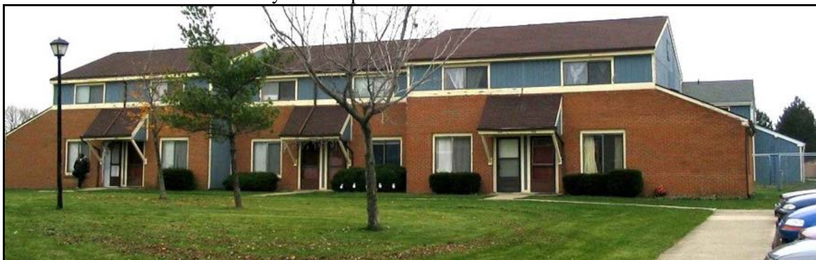
Liberty Plaza Apartments Prior to Rehabilitation
