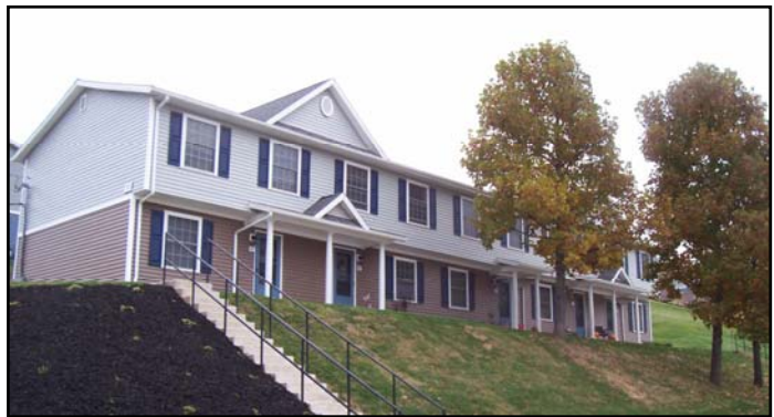
Powell Apartments after Rehabilitation
