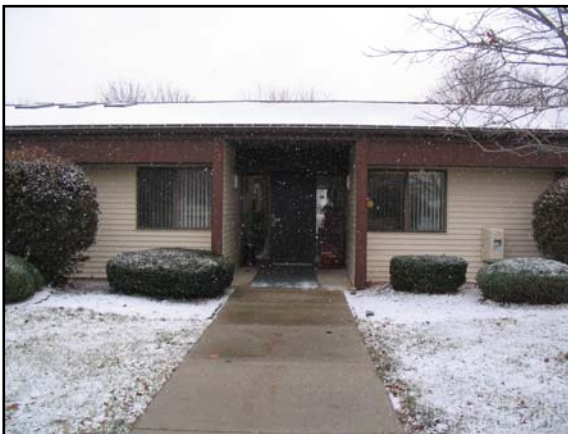
Hinman-Smith Prior to Rehabilitation
