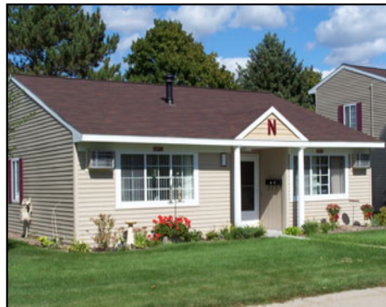
Hinman-Smith Subsequent to Rehabilitation
