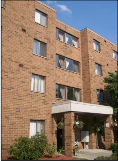
Highland Place Apartments Prior to Rehabilitation
