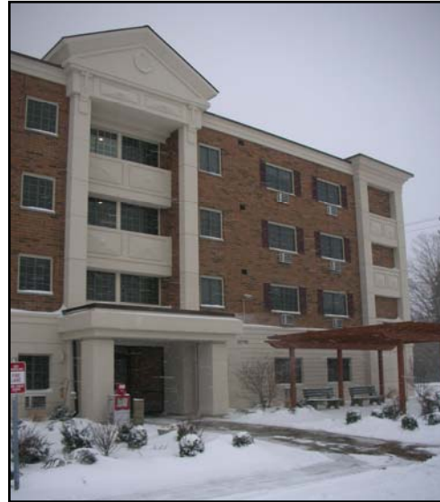
Highland Place Apartments Subsequent to Rehabilitation
